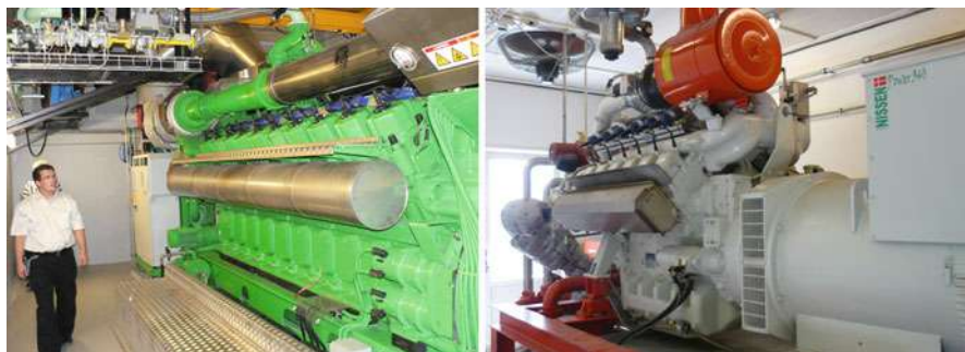
Fig. 35 Snedsted CHP ( left ) with GE Jenbacher V20 3,500 kWel gas motor. Farm CHP ( right ) with MAN V12 375 kWel motor using biogas (Preben Maegaard/Nordic Folkecenter for Renewable Energy)
