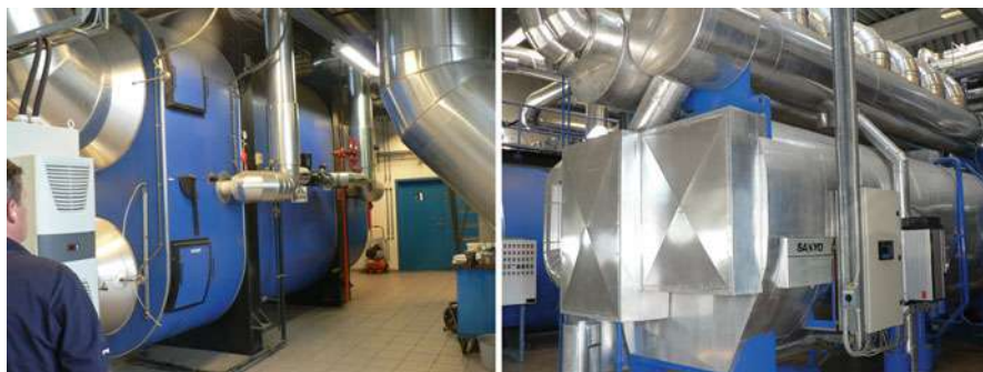
Fig. 34 Ancillary equipment in a CHP station: the exhaust heat exchangers ( left ) convert the exhaust heat from the gas engines to hot water. The absorption heat pump ( right ) upgrades 20–40 °C water for use in district heating (Preben Maegaard/Nordic Folkecenter for Renewable Energy)
