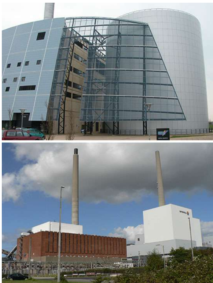
Fig. 18 Viborg CHP plant ( Top ) using natural gas turbine for the production of heat and electricity. The hot water storage is seen to the right of the turbine hall. The city of Odense ( Bottom ) with its 165,000 inhabitants was a pioneer within large urban CHP resulting in low heating costs. Fuels for the supply of steam to the turbines are straw, household waste, and natural gas (Preben Maegaard/Nordic Folkecenter for Renewable Energy)
