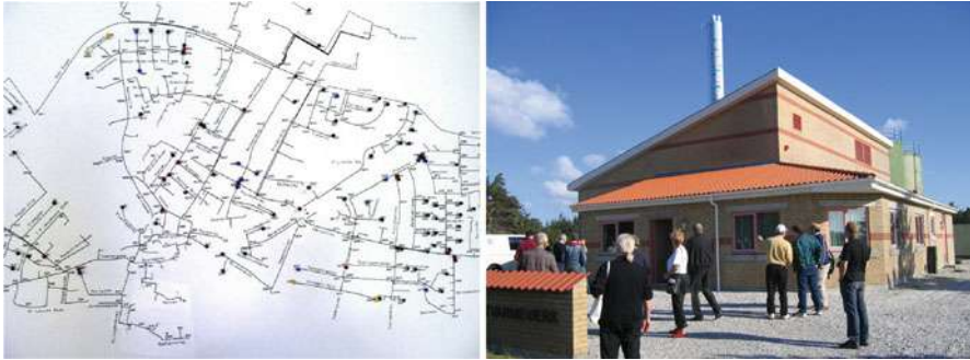
Fig. 40 Example of a district heating network ( left ). Vorupoer CHP ( right ) has two Jenbacher natural gas motors, each of 900 kWel. The electrical efficiency is 42 %. It serves 200 households, local business, and institutions with heat. The electricity is delivered to the public grid. The chimney is decorated by a local artist. In the background are two hot water storagetanks. The CHP and heating network is owned by the local consumers in a not-for-profit company. The staff consists of one person, a technician. In 2010 the plant was presented in the film documentary “The 4th Revolution” as an example of best practice (Jane Kruse/Nordic Folkecenter for Renewable Energy)
