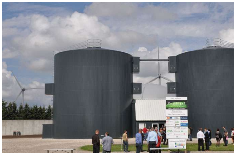
Fig. 50 Farm biogas plant of the ComBiogas type during the inauguration. Through a network of pipes the slurry is pumped from the farms for digestion and returned back for spreading as fertilizer over the fields. The biogas is piped to the nearest CHP station (Jane Kruse/Nordic Folkecenter for Renewable Energy)
