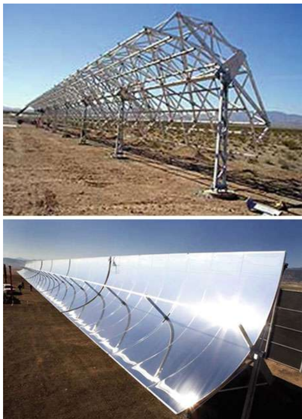
Fig. 8 Left: parabolic trough space frame structure (Source: NREL). Right: lightweight trough with reflective thin film mirror (Farr and Gee 2009)
