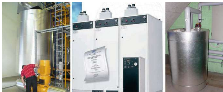
Fig. 46 Three sizes and types of electric boilers for power downregulation: 20 MW, 10 kV ( left ); 3,300 kW, 400 V ( middle ); and 45 kW, 400 V ( right ) (Nordic Folkecenter for Renewable Energy)
