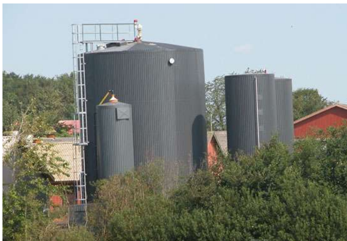
Fig. 53 Biogas plant at farm in Denmark. The gear motor for the internal slow-moving agitator is seen on top the digester (Jane Kruse/Nordic Folkecenter for Renewable Energy)
