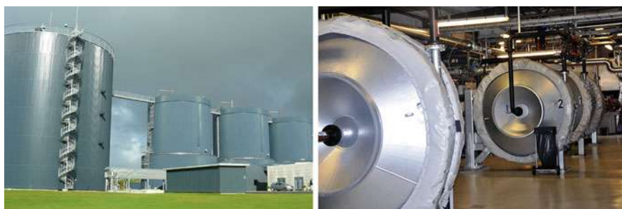
Fig. 58 Left: Lemvig Biogas Plant (Jane Kruse/Nordic Folkecenter for Renewable Energy). Right: Slurry-to-slurry heat exchangers at Lemvig Biogas Plant reduce the demand for process energy for heating the digesters (Jane Kruse/Nordic Folkecenter for Renewable Energy)
