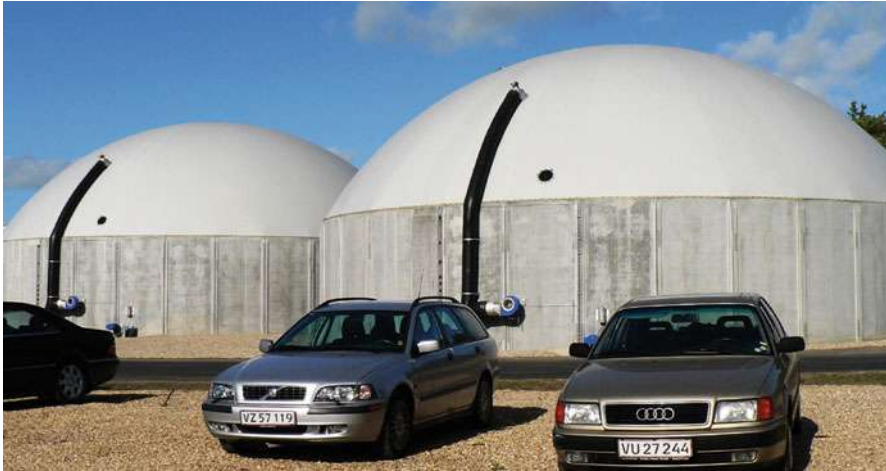
Fig. 54 Biogas storage tanks at community plant (Preben Maegaard/Nordic Folkecenter for Renewable Energy)
