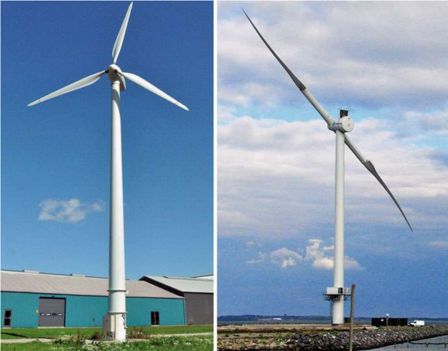
Fig. 27 (Left) 25 KW solid wind of the new household wind turbine generation for single families and farms. Production: 40,000–80,000 kWh per year. (Right) Envision 3 MW wind turbine prototype during testing in Thyborøn, Denmark. Engineering and design by a Chinese company’s R&D division in Denmark (Preben Maegaard/Nordic Folkecenter for Renewable Energy)
