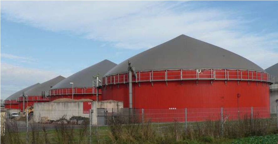
Fig. 55 Big farm biogas plant on the island of Rügen, Germany. In Germany there are several thousands of farm biogas plants with digestion of animal manure and energy crops. The biogas is normally combusted in gas engines on location (Preben Maegaard/Nordic Folkecenter for Renewable Energy)
