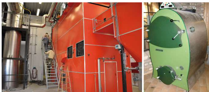
Fig. 20 Large scale: Boiler for wood chips in district heating station for town with 4,000 residents (left). Small scale: Hertl boiler, capacity up to 145 KW th , for the gasification of especially wood stems (right) (Jane Kruse/Nordic Folkecenter for Renewable Energy)
