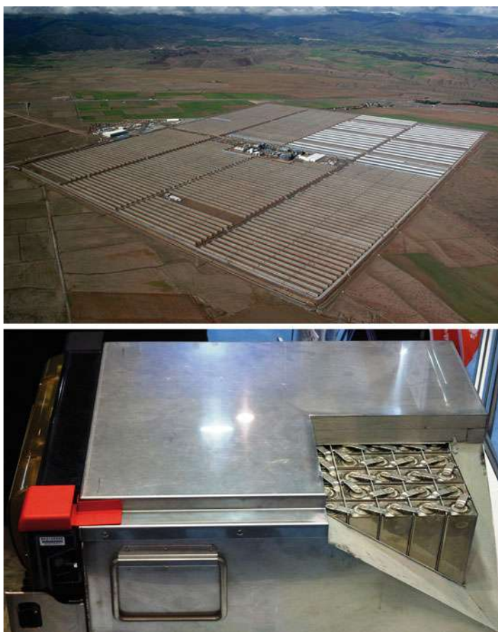
Fig. 16 The 150 MW Andasol solar power station ( Top ) is a commercial parabolic trough solar thermal power plant, located in Aldeire, Granada, Spain. The Andasol plant uses tanks of molten salt to store solar energy so that it can continue generating electricity even when the sun is not shining (BSMPS). ( Bottom ) Molten salt secondary battery (FIAMM SoNick) (Rudolf Simon)
