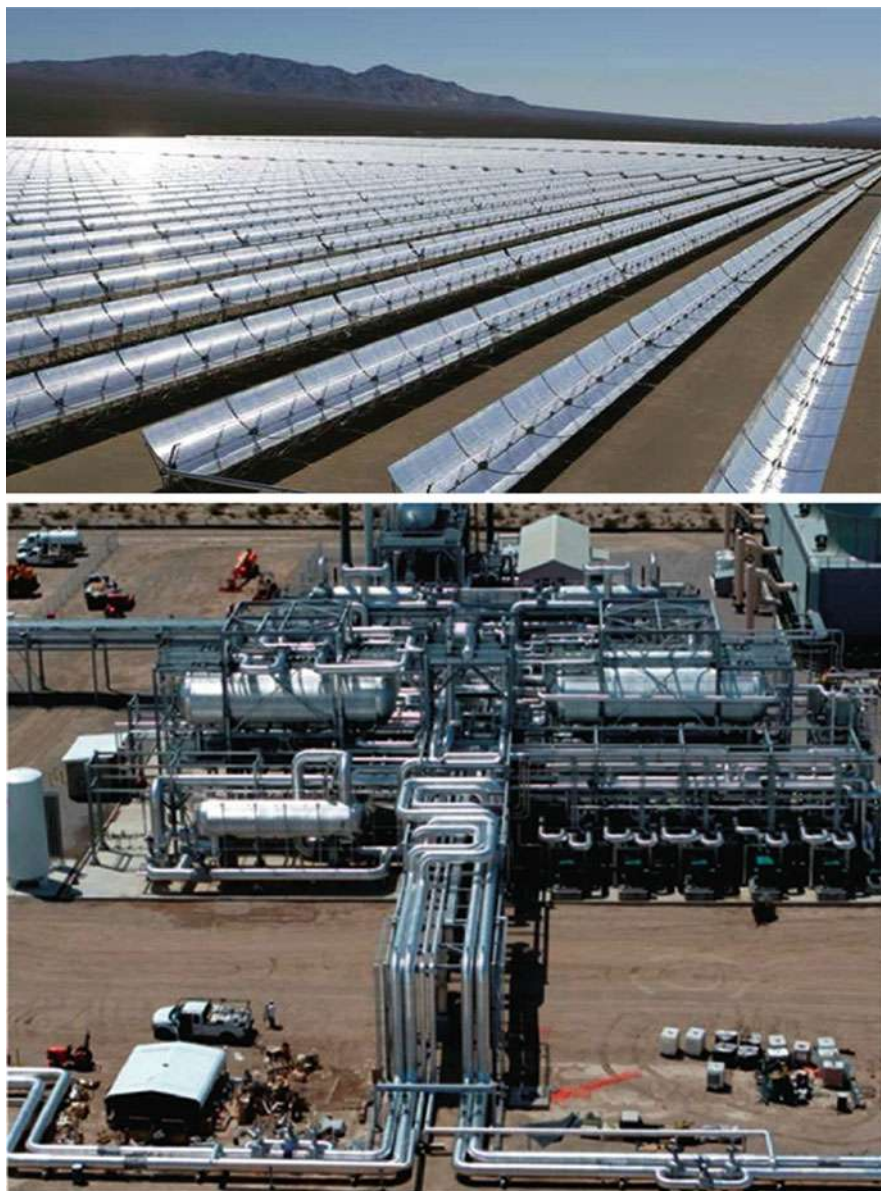
Fig. 12 Left: parabolic trough field. Right: power block at Nevada Solar One power plant (Source: www.acciona-na.com )
