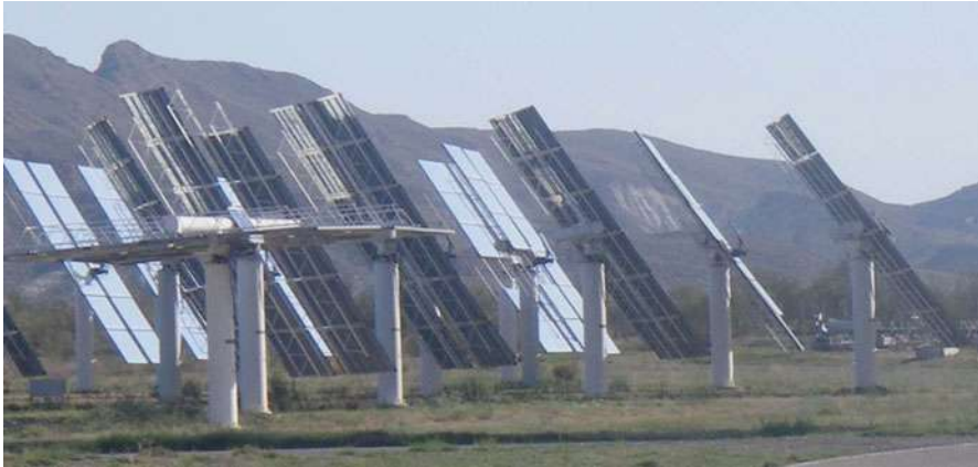
Fig. 24 Typical advanced heliostat field (Source: Plataforma Solar de Almeria – PSA, Spain)
