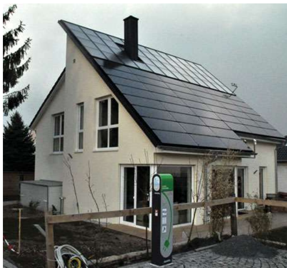
Fig. 4 Energy autonomous house in Freiberg, Germany. Gray battery electricity storage box and its own car charging station (Preben Maegaard/Nordic Folkecenter for Renewable Energy)
