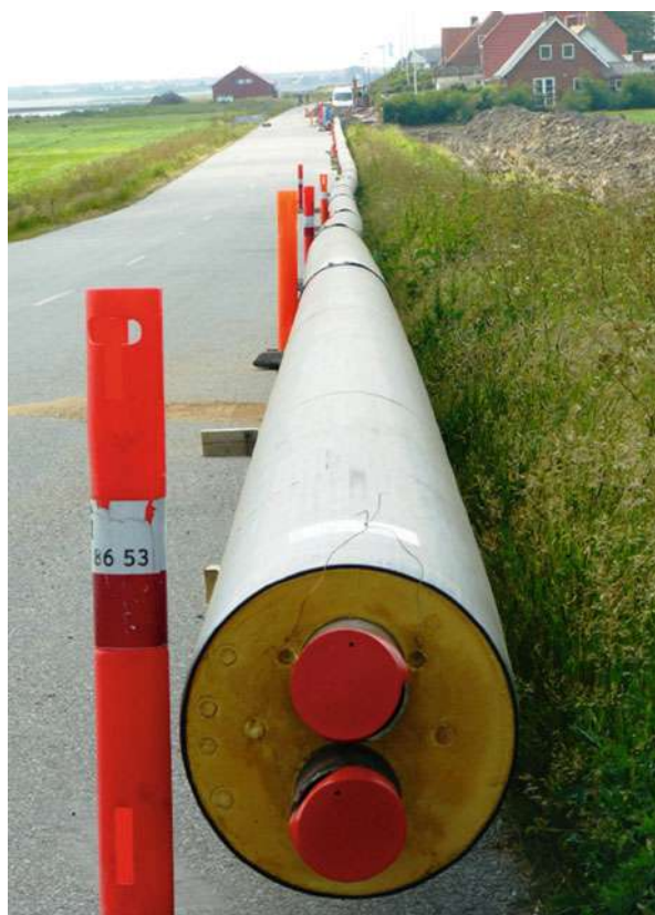
Fig. 41 PU foam insulated pipes ( left ) for district heating for a small rural community (Preben Maegaard/Nordic Folkecenter for Renewable Energy). ( right ) Through well-insulated heating pipes (red), 60–90 °C water is circulated to every building. After cooling down to approximately 30–50 °C, the water returns (blue) to the CHP station (Jane Kruse/Nordic Folkecenter for Renewable Energy)
