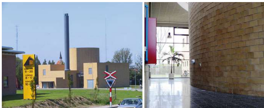
Fig. 33 Faaborg CHP plant ( left ) with its location close to the town center. It can supply its 7,000 inhabitants. The circular center building is for the hot water storage ( right ) (Jane Kruse/Nordic Folkecenter for Renewable Energy)
