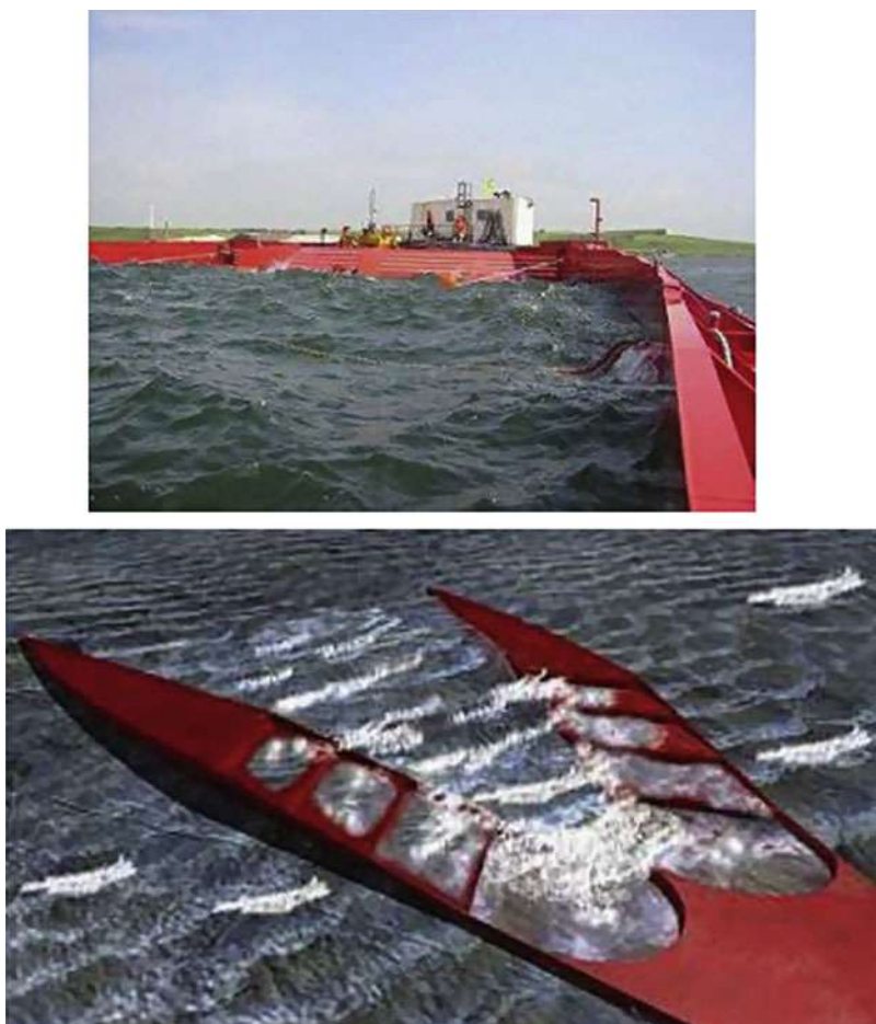
Fig. 8 Overtopping wave energy converters: Wave Dragon ( top ) and WaveCat ( bottom ) (Courtesy of Wave Dragon AS (2005) and the COAST Research Group at Plymouth University and Fernandez et al. (2012))
