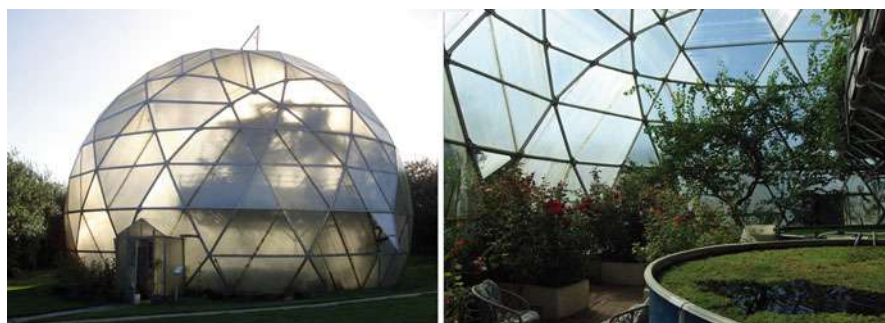
Fig. 67 Dike-pond system in the biodome, Nordic Folkecenter for Renewable Energy. The biodome is a unique greenhouse, which integrates water cycle, recycling of nutrients, insulation, and aquaculture (Anna Krenz/Nordic Folkecenter for Renewable Energy)
