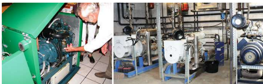
Fig. 36 Two types of small-scale CHP in Bavaria, Germany. KW Energie CHP ( left ) with Kubota 8 kWel/18 kWth engine for one family house using pure plant oil, PPO. Farm CHP ( right ) with 3 \times 120 kWel (approx.) MAN engines using biogas (Preben Maegaard/Nordic Folkecenter for Renewable Energy)
