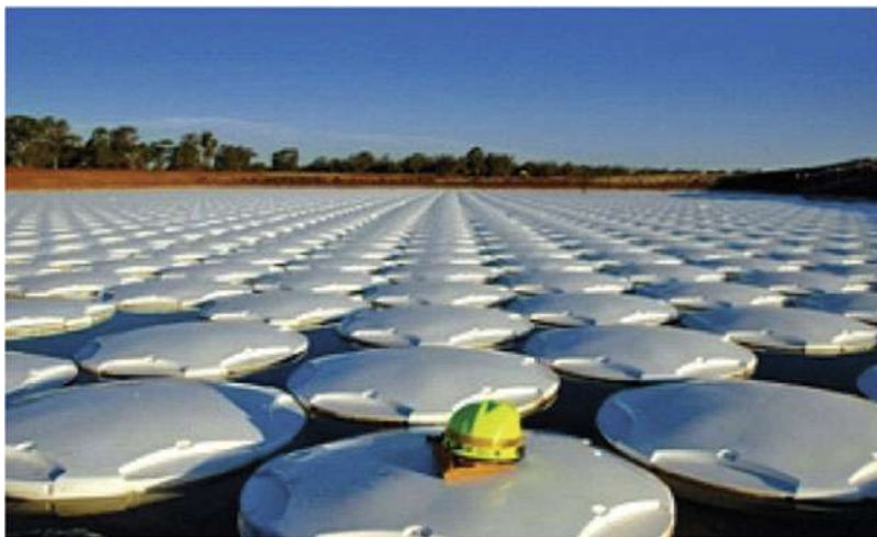
Fig. 7 Reflective evaporation covers on a mine reservoir at Parkes in Australia (Edmonds and Smith 2011)
