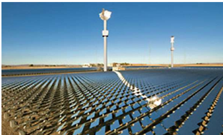
Fig. 27 5 MW twin central receiver tower facility with 1 m 2 heliostats in California (Source: eSolar)
