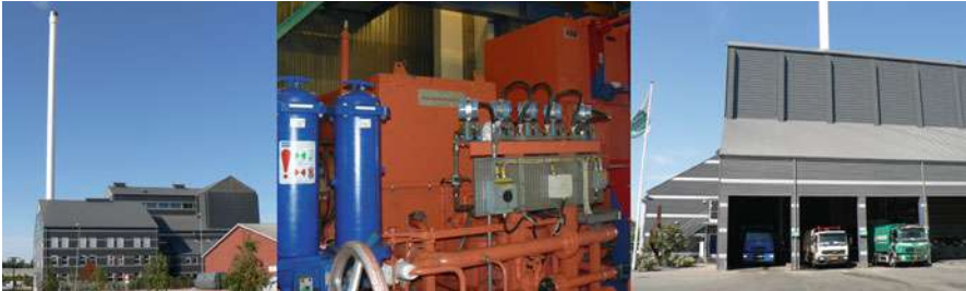
Fig. 47 (Left) Thisted combined heat and power for a town of 25,000 residents. Fuels used include household waste, straw, wood, solar thermal, and geothermal. (Middle) 6 MWel steam turbine. (Right) trucks discharge waste (Jane Kruse/Nordic Folkecenter for Renewable Energy)
