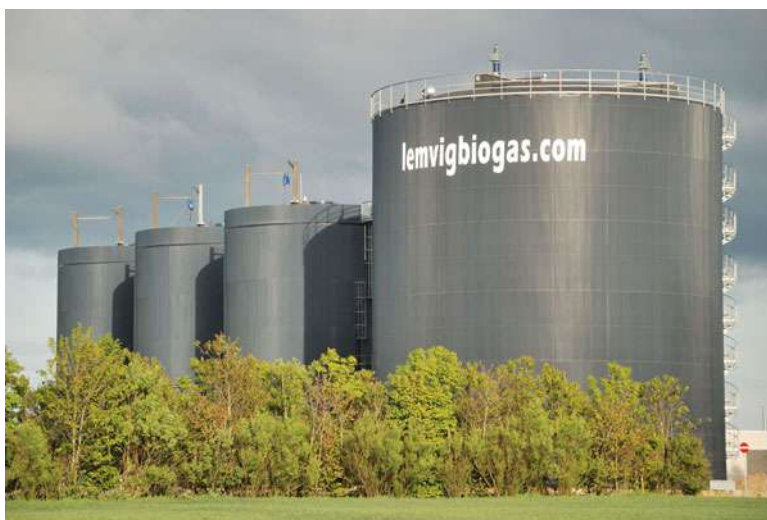
Fig 57 Reactor tanks of 14,300 m 3 at the Lemvig Biogas Plant (Photo: lemvigbiogas.com)
