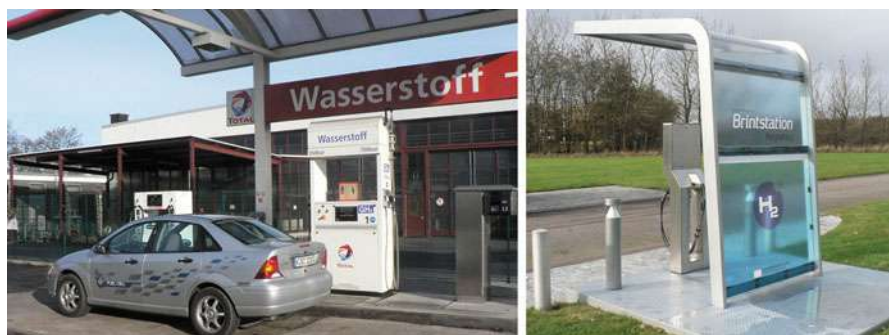
Fig. 64 (Left) Fuel cell car at hydrogen filling station at major radial road, Berlin, Germany. (Right) Compact hydrogen filling station for cars and vans in Ringkøbing, Denmark. Developed by H2 Logic (Preben Maegaard/Nordic Folkecenter for Renewable Energy)
