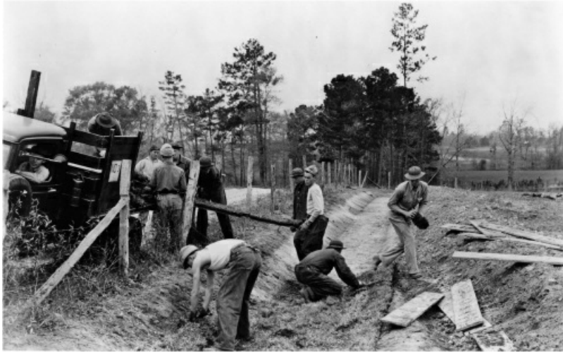
Figure 7 Soil Conservation Service. CCC workers putting sod along a gulch to prevent soil erosion. Courtesy: FDR Library
